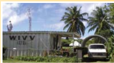
Mark Freed (from EWO) on top of a radio station appraising the maintenance of the tower and roof.
